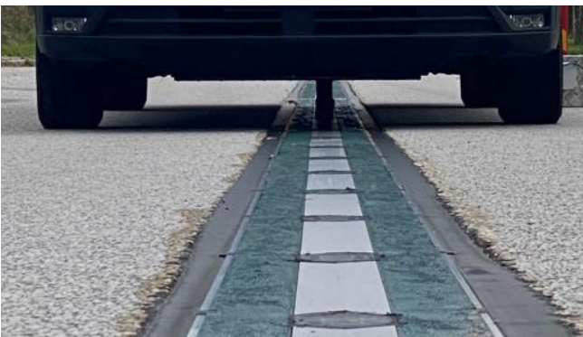
Figure 2. Elonroad conductive in-road rail
