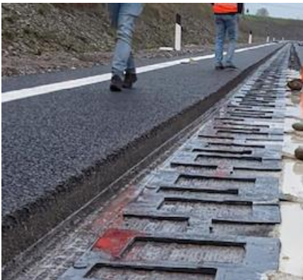
Figure 5. Inductive embedded coils, wireless ERS
